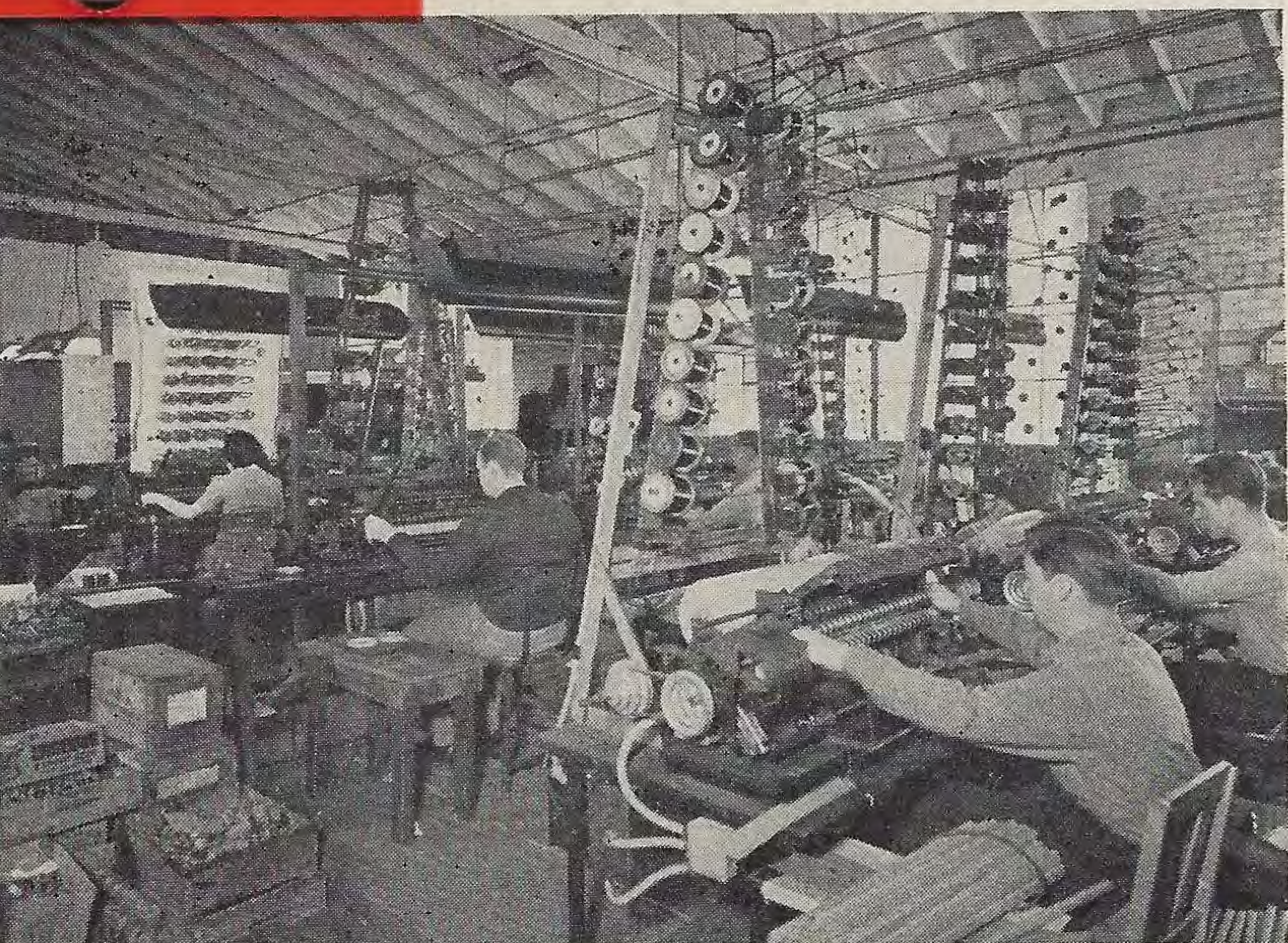
Transformer coils in groups of from 5 to 40, are wound at one time on semi-automatic winding machines of Peerless design.
