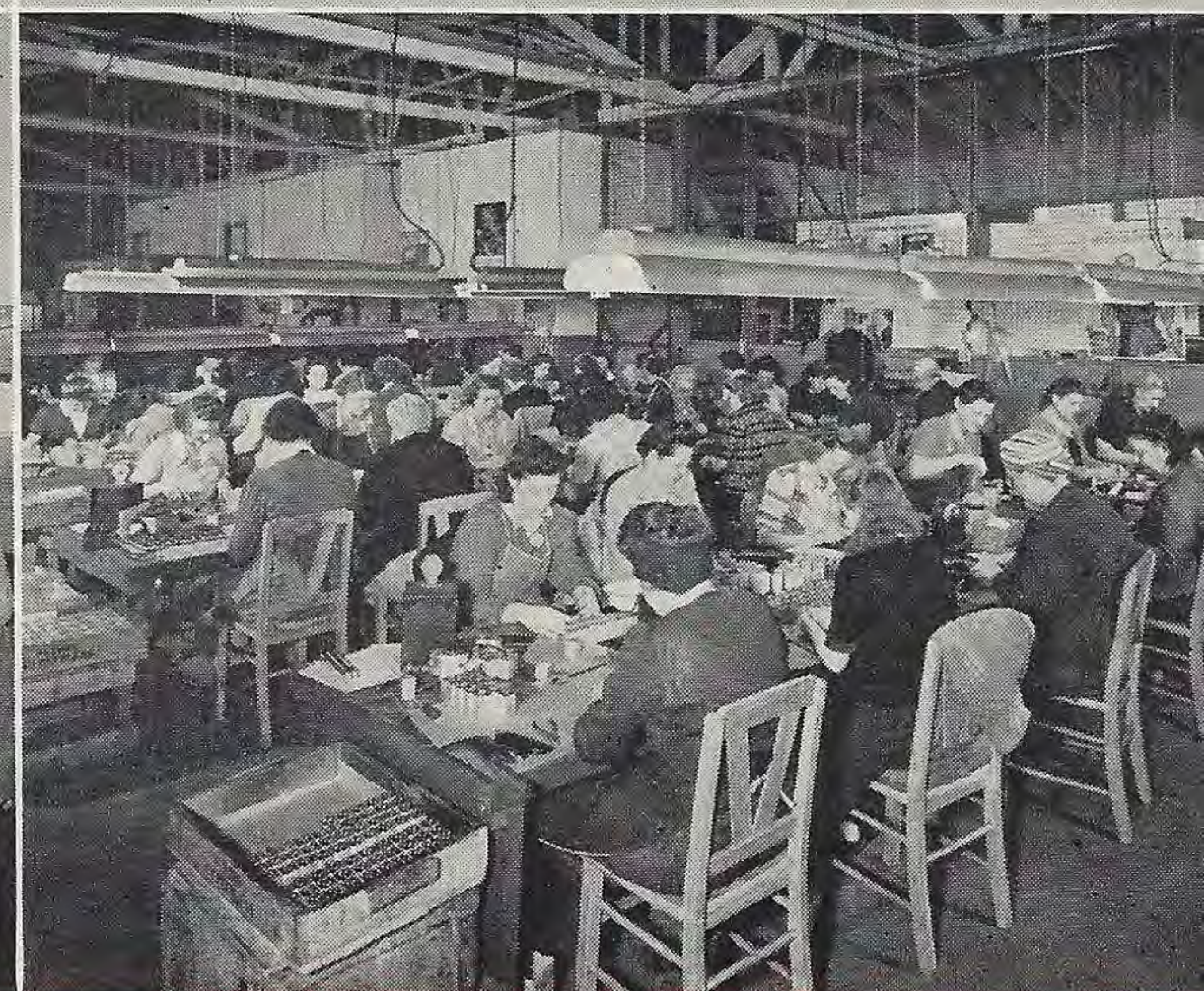
Final assembly department for Peerless transformers—the last stage before testing. Various sizes and forms of transformers can be noted.
